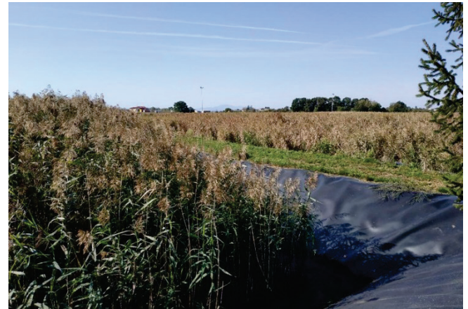
Figure 4 Constructed reed beds within WWTP Cakovec
