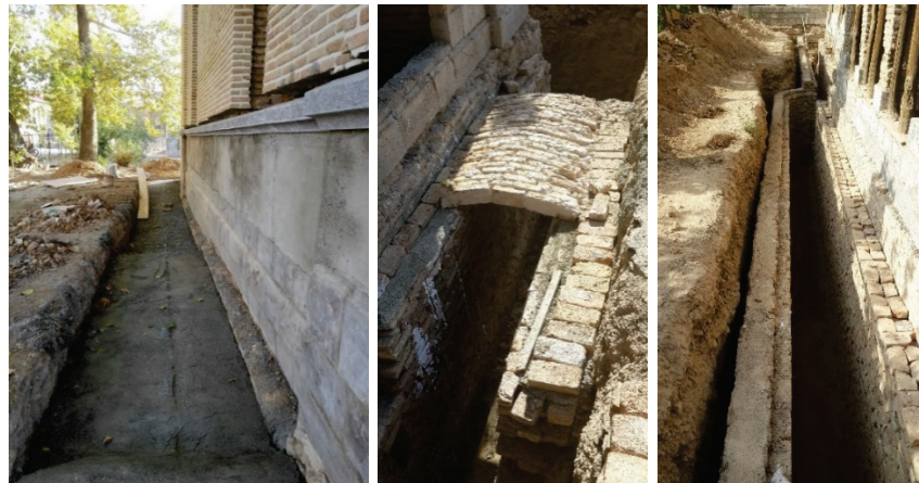
Figure 6 Images of the construction of building No. 4, University of Arts, National garden Campus, Source: (Technical Department and Supervision of Development Plans of the University of Arts) 1400
