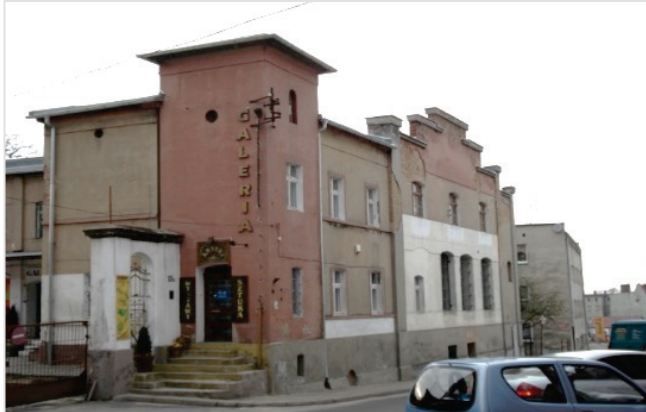
Figure 1 Elevation facing Fabryczna St. (first section) prior to adaption
