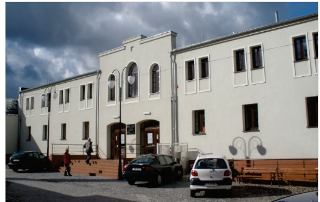
Figure 4 Southeast elevation of building (second part) after adaption
