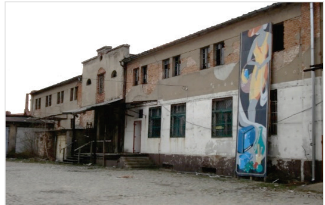
Figure 3 Southeast elevation of building (second part) prior to adaption
