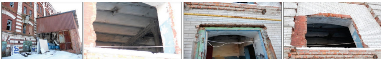
Figure 2 Physical conditions of the building
