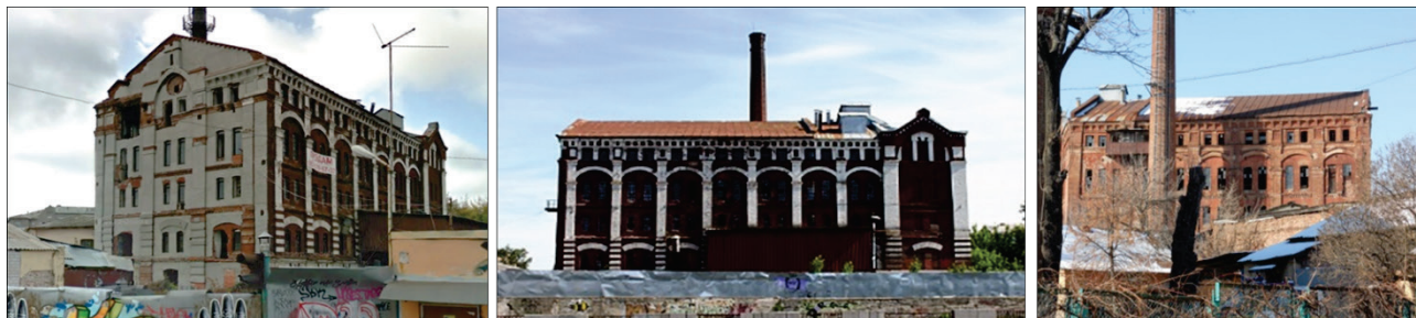
Figure 1 The old mill building
