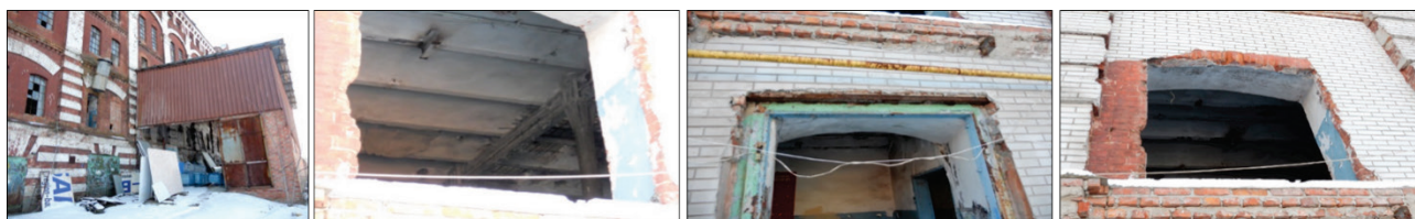
Figure 2 Physical conditions of the building
